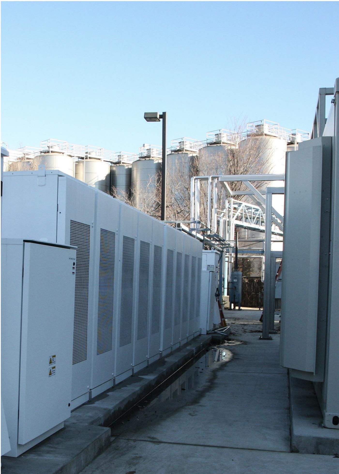
*The 1 megawatt-hour of Powerpack batteries holds enough energy to drastically reduce the brewery's demand charges. (Photo credit: Sierra Nevada)*
