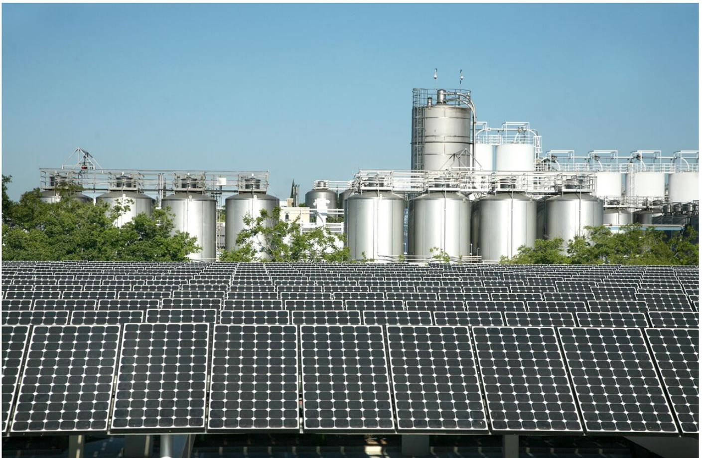
*Sierra Nevada's 10,751 solar modules generate 2 megawatts of power and offset 20 percent of the brewery's annual electricity consumption. (Photo credit: Sierra Nevada)*
